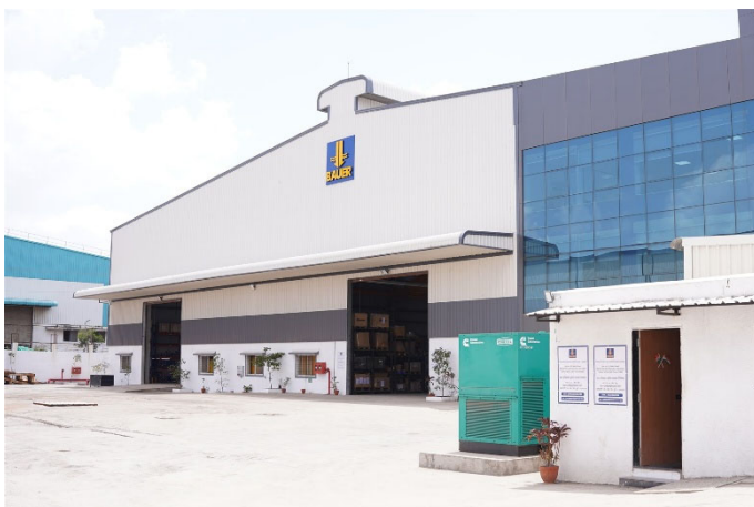
(3) Exterior view of the BAUER Maschinen facility in Pune
